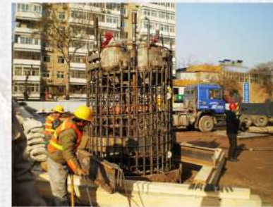
Install the rebar cage
