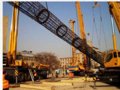
Lift the cage with Super Cell
