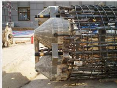
Weld Super Cell to the cage
